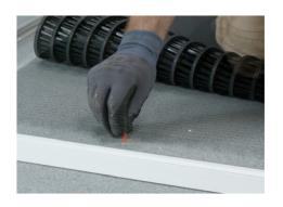
Fix the aluminum frame to the floor with screws.
