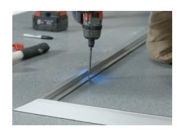
Position one end of the mat under the edging strip and lay in the aluminum frame.
