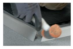
When completing the final side of the frame, make sure you fit both inserts into the single remaining edge.
