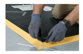
Apply cold weld paste to the PVC edging to connect the edging to the matting. The base bar should sit flush to the edge. Apply weights and allow to dry for **30 minutes**. Repeat on each edge.
