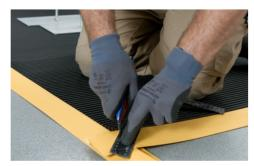
Apply cold weld paste to the mitered edge.
