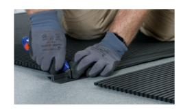
On one side of the snap track, apply cold weld paste to the full length of the snap track then press mat in place. Apply weights and leave to dry for **30 minutes**.
