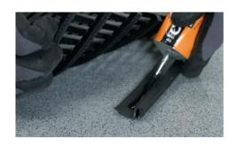
Trim any protruding base bars so the snap track sits flush. On the second part of the snap track, apply cold weld paste and press the mat in place. Apply weights and leave to dry for **30 minutes**.
