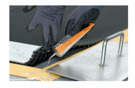
Carefully bend back the edging and fill the gaps with cold weld paste.
