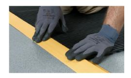
To make the corner, miter the PVC edges at a 45-degree angle. Use a straight edge and a sharp utility knife to the cut.
