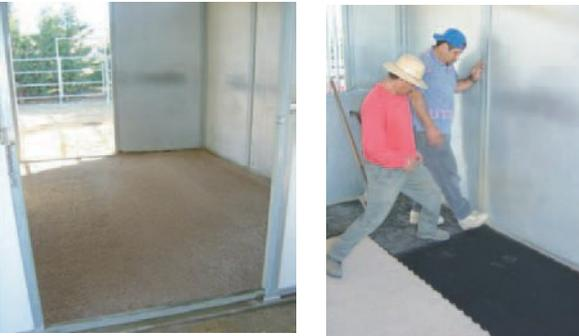
Now that the subsurface is level and compacted, let it dry and you are ready to install the mats. Using the stall diagram, the mats are marked on the bottom with numbers from the diagram. Start in one corner of the stall and fit pieces together like puzzle, once the interlock is started, you can walk over them to fit in place. Because rubber can expand and contract, we recommend that you leave a 1/4" to 1/2" gap between the edge of the mat and the stall wall.
