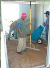
**Step 2-** use 3/4" board (mat thickness) to make sure you have enough fines for stall elevation
