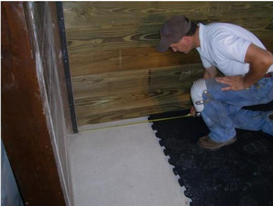
**Step four** is to mark your mat for cutting. Measure your mat from the male end of an interlocking tab. The more detailed you can mark your mat; the less opportunity there is to make a mistake. Use the BIC White-Out pen to "sketch" your cuts out on the stall mat. It is also a good idea to take a moment and re-check your measurements before you begin cutting. Remember: MEASURE TWICE - CUT ONCE!
