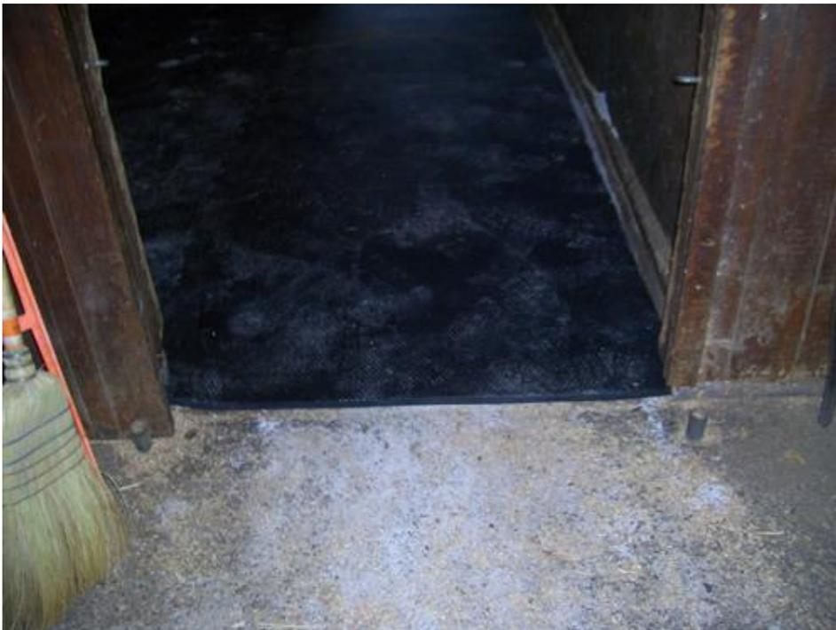
A properly installed doorway mat should extend out and tightly butt up against the stall door or threshold.
