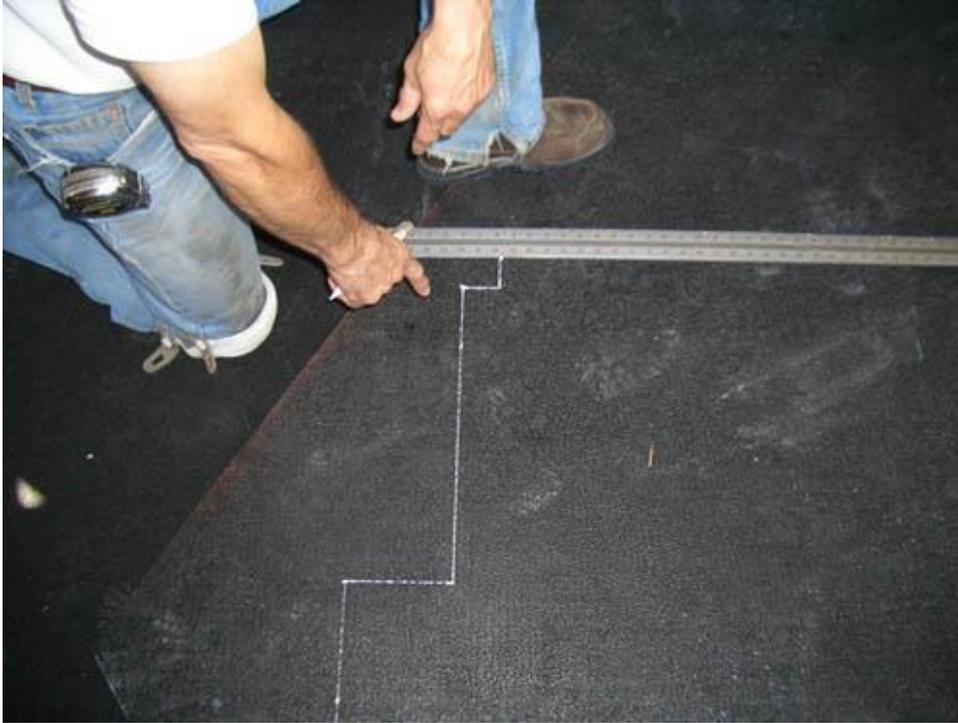
After you have your mat "sketched" out, it is time to begin cutting. Place your "T" square along the line to be cut. Put the blade of your utility knife along the edge of the "T" square and using it as a guide, begin scoring the line to be cut with your knife. Score this line 3 to 5 times until you have cut over half way through the rubber.
