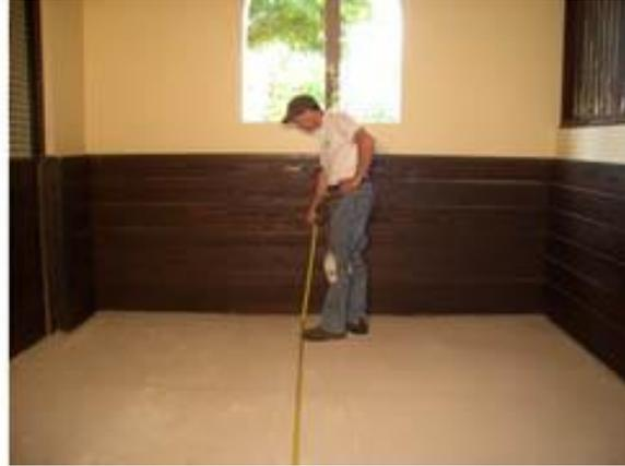
Measuring first will prevent you from making costly mistakes later. A properly installed stable floor should run wall to wall and fit as tight as possible. The key is to build large and cut to fit.
