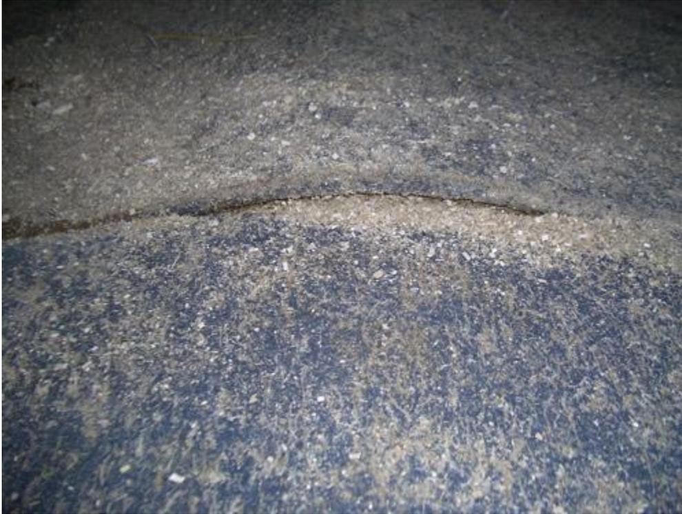
Here is an example of the type of damage that a horse can do to an improperly installed stable floor. This matting was laid over the uneven dirt base previously pictured.
