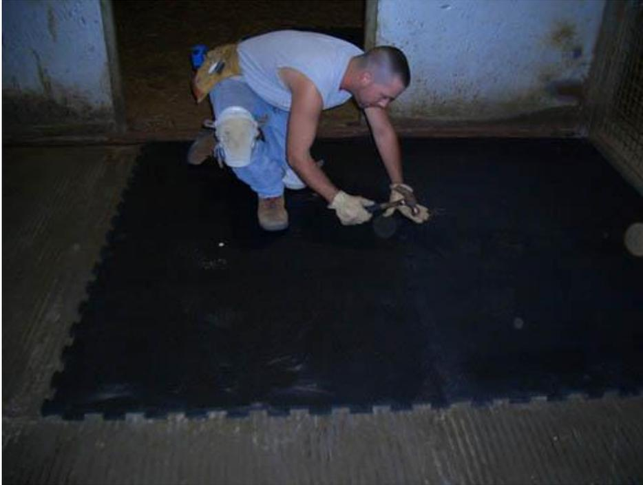
You will now want to measure from the female end of an interlocking tab on the mat over to the furthest point on the wall. Take a measurement from both the top and the bottom edges of the mat. (This will tell you if your wall is out of square.) Take notice of any objects or protrusions that will need to be cut around. (posts, etc.)
