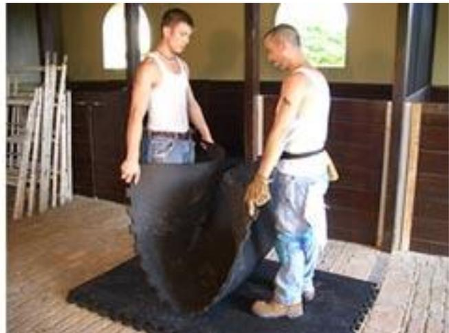
Notice how these installers have folded the mat in half and are grabbing it by the corners. They then put their knees into the mat to bow it away from themselves. Finally, they lift the mat from the ground. This "bowing" technique will not only make it easier to move the mat through the stall door, but greatly reduces the amount of weight put on the individuals carrying the mats.
