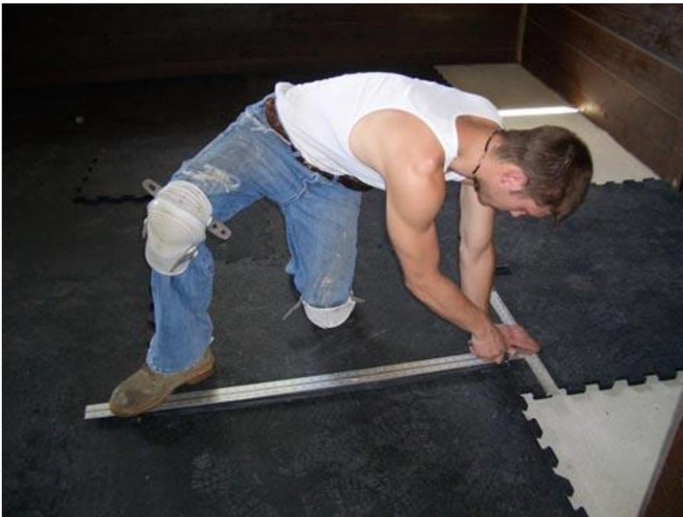
Note the position of the installer's hands and feet. You can either use your foot or knee to hold the end of the "T" square in place. Your free hand should always be towards the top of the "T" square and out of the way of the knife's blade.
