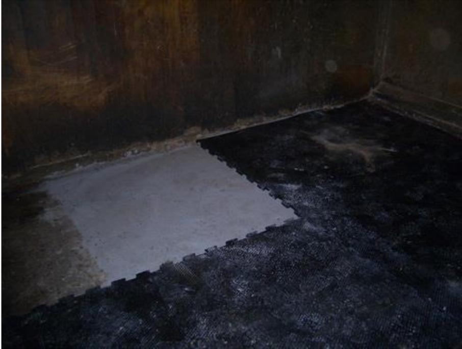
By creating this "L" shape you have given yourself points from which you can measure in both directions. This is an important step in fitting your last mat tightly into the doorway of the stall.
