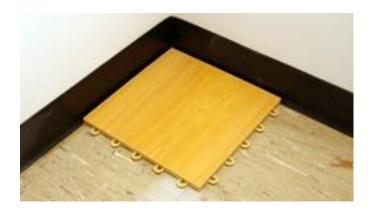
**Step 3** Place the next panel so that the pegs line up over the loops:
