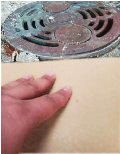
Fixture too high; ramping required
