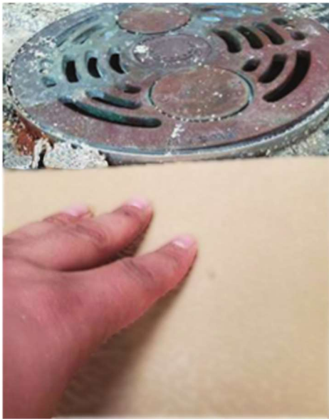
Fixture too high; ramping required
