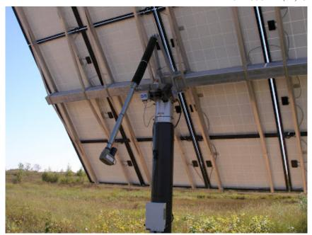
These PV arrays are equipped with gears and motors that allow the panels to remain oriented toward the sun throughout the day and across the seasons. Called a dual axis tracking system, this feature significantly boosts power output.
