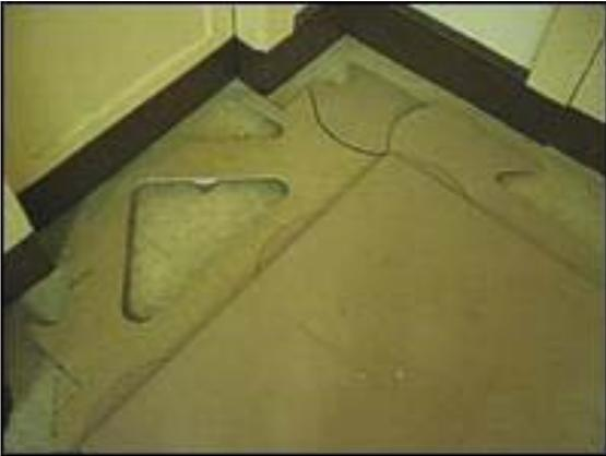
Customizing Panels filling corner of room right to the wall. Note the small infill to make up the corner. The MDF filler will support the small corner piece.
