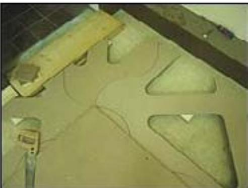
Customizing Panels making up corner with doorway. Note leveling shims in place to level floor. Also note 2" x 6" which will support ramp in doorway.
