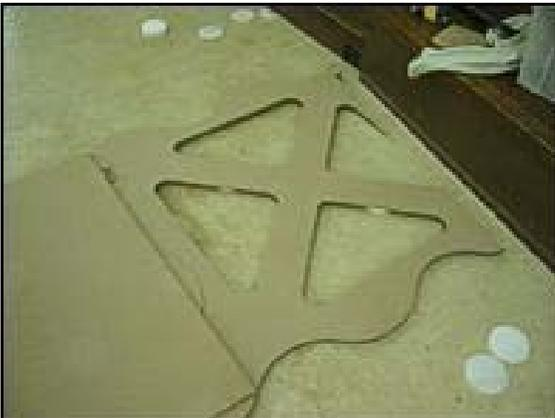
Customizing Panel cut with curve of stage. Panel is cut 4" from wall. A 2" x 4" is placed against the wall and the whole surface is finished with MDF screwed to the Customized Panels and to the subfloor panel.
