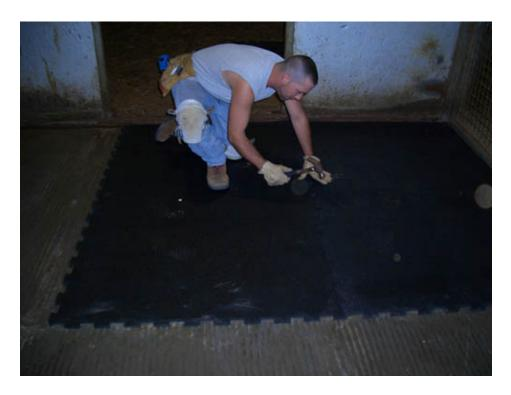
You will now want to measure from the female end of an interlocking tab on the mat over to the furthest point on the wall. Take a measurement from both the top and the bottom edges of the mat. (This will tell you if your wall is out of square.) Take notice of any objects or protrusions that will need to be cut around. (posts, etc.)
