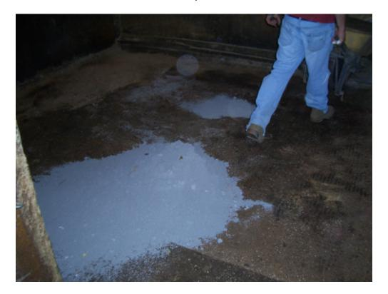
The stone dust can be brought into the stall using a front-end loader or a wheelbarrow.
