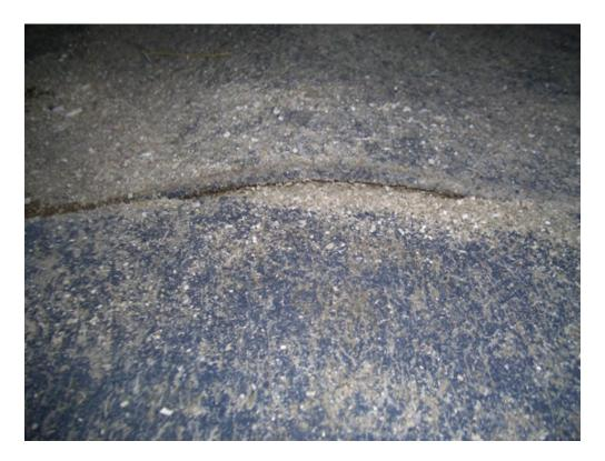
Here is an example of the type of damage that a horse can do to an improperly installed stable floor. This matting was laid over the uneven dirt base previously pictured.
