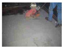
A finished sub-floor should be hard, smooth, and level. You should be able to walk across it without leaving a footprint.
