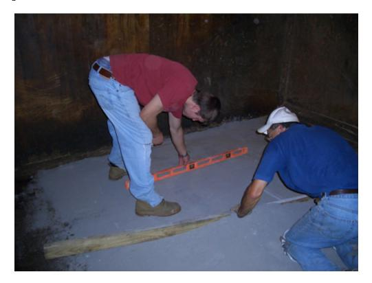
Check your sub-floor to make sure you are spreading the stone dust evenly and level.
