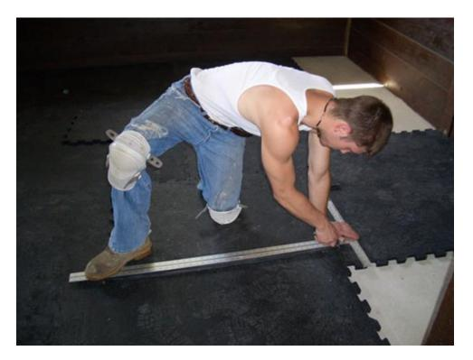
Note the position of the installer's hands and feet. You can either use your foot or knee to hold the end of the "T" square in place. Your free hand should always be towards the top of the "T" square and out of the way of the knife's blade.
