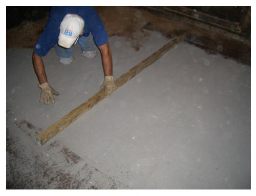
Using an old 2'x 4' to help spread the stone dust will also show you if there are any low spots in the floor where you might need to add more of the crushed stone base.
