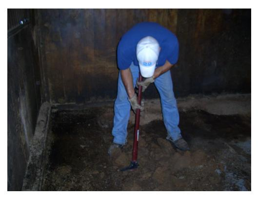
Once the dirt floor has been leveled, it is time to bring in the stone dust. The stone dust should be spread evenly across the stall floor about 4 to 6 inches deep.
