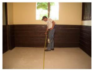
Measuring first will prevent you from making costly mistakes later. A properly installed stable floor should run wall to wall and fit as tight as possible. The key is to build large and cut to fit.
