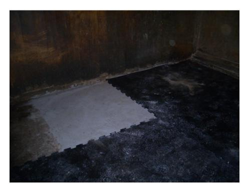
By creating this "L" shape you have given yourself points from which you can measure in both directions. This is an important step in fitting your last mat tightly into the doorway of the stall.
