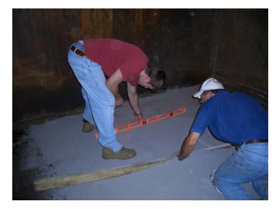
Check your sub-floor to make sure you are spreading the stone dust evenly and level.
