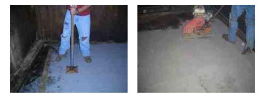
A finished sub-floor should be hard, smooth, and level. You should be able to walk across it without leaving a footprint.
