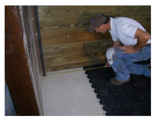
**Step four** is to mark your mat for cutting. Measure your mat from the male end of an interlocking tab. The more detailed you can mark your mat; the less opportunity there is to make a mistake. Use the BIC White-Out pen to "sketch" your cuts out on the stall mat. It is also a good idea to take a moment and recheck your measurements before you begin cutting. Remember: MEASURE TWICE - CUT ONCE!
