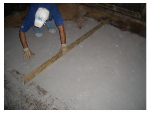
Using an old 2'x 4' to help spread the stone dust will also show you if there are any low spots in the floor where you might need to add more of the crushed stone base.
