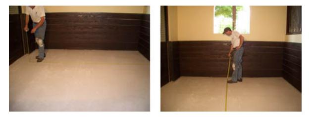
Measuring first will prevent you from making costly mistakes later. A properly installed stable floor should run wall to wall and fit as tight as possible. The key is to build large and cut to fit.
