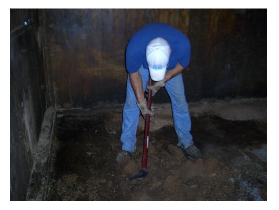
Once the dirt floor has been leveled, it is time to bring in the stone dust. The stone dust should be spread evenly across the stall floor about 4 to 6 inches deep.
