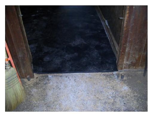
A properly installed doorway mat should extend out and tightly butt up against the stall door or threshold.
