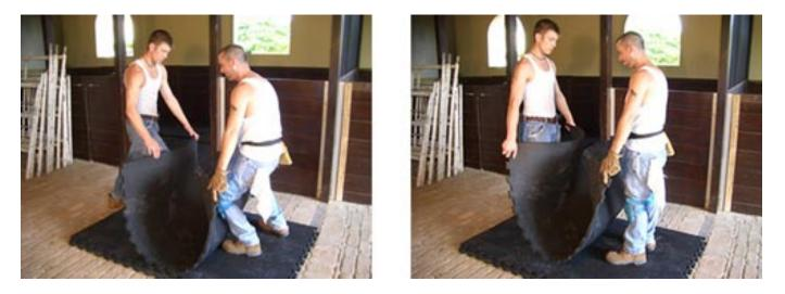
Notice how these installers have folded the mat in half and are grabbing it by the corners. They then put their knees into the mat to bow it away from themselves. Finally, they lift the mat from the ground. This "bowing" technique will not only make it easier to move the mat through the stall door, but greatly reduces the amount of weight put on the individuals carrying the mats.
