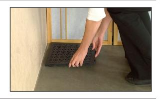
2. Keeping all additional tiles facing in the same direction, place tabs of new tiles over loops of already laid tiles and push down until they pop into place.
