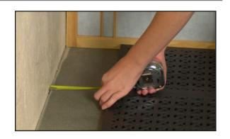
2. Using pen or marker, mark that distance on the tile you'd like to cut, keeping in mind direction of the tile.
