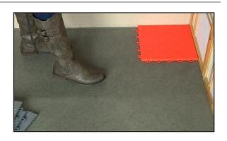
2. Keeping all additional tiles facing in the same direction, place tabs of new tiles over loops of already laid tiles and push down until they snap into place.
