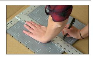
4. Cut along lines using power saw OR cut halfway through with the sharp utility knife using a series of shallow scores and fold back at cut until it breaks.
