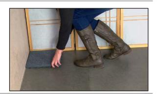
2. Keeping the loops in the same direction, continue to add tiles, alternating the orientation or grain of the carpet with each tile, creating a checkerboard pattern. Place tabs of new tiles over loops of the already laid tiles and push down until they snap into place.
